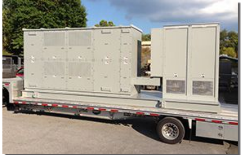
Shown above: 15kV Substation Style 2500kW Load Bank
